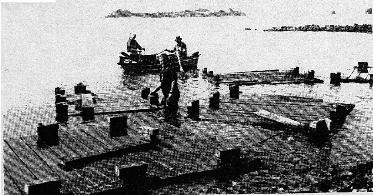
Sections of the dismantled jetty are floated across the bay.
